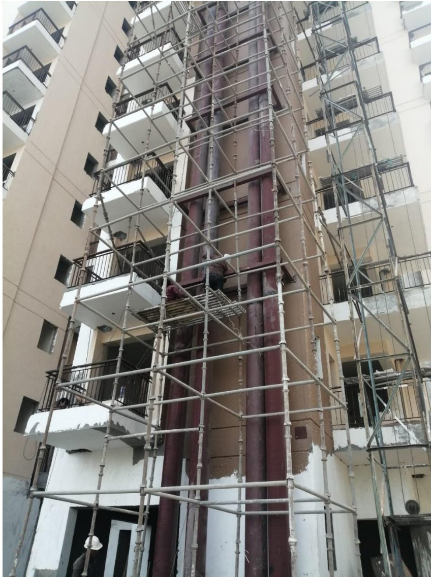
DG Stack Work is in Progress
