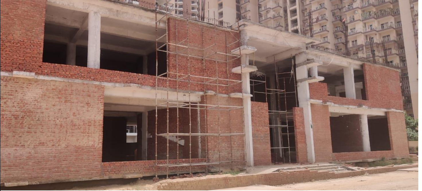
School Finishing work is in progress
